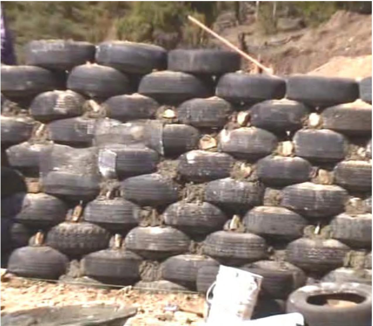
The tyres are overlapped in successive rows, forming a stable structure and then grouting is applied between them. The outside is enclosed in an earth bank and the inside is later smoothed over.
